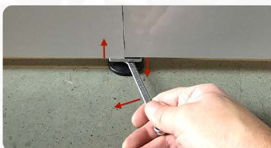
PANEL ALIGNMENT WITH MIO WRENCH
