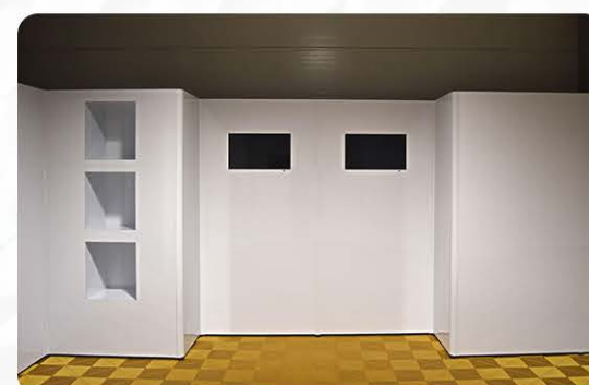
FINAL PANELING OF THE COMPOSITE BOARDS ON MAGTAPES
